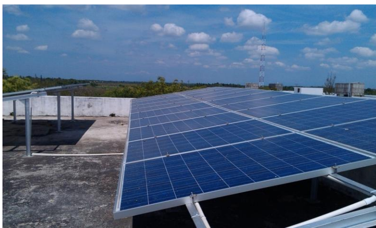
MNRE Sponsored 25KW solar power generation system at Admin Block
